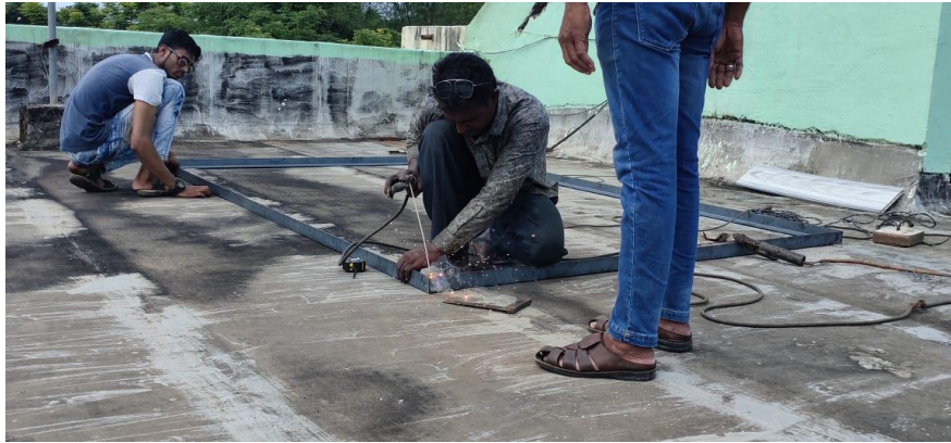
SHIELDED ARC WELDING OF THE FRAME
