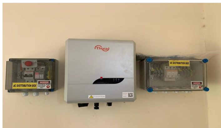
(FROM LEFT TO RIGHT) AC DISTRIBUTION BOX, SOLAR INVERTER, DC DISTRIBUTION BOX
