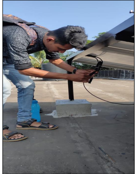
Connecting Solar panels in series
