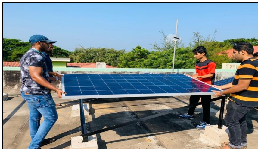
Mounting a solar panel
