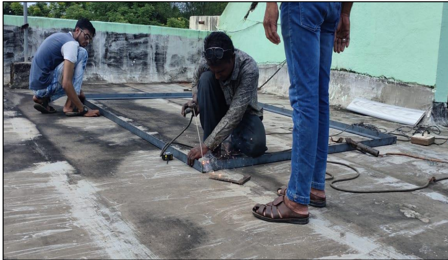
Shielding Arc welding of the frame
